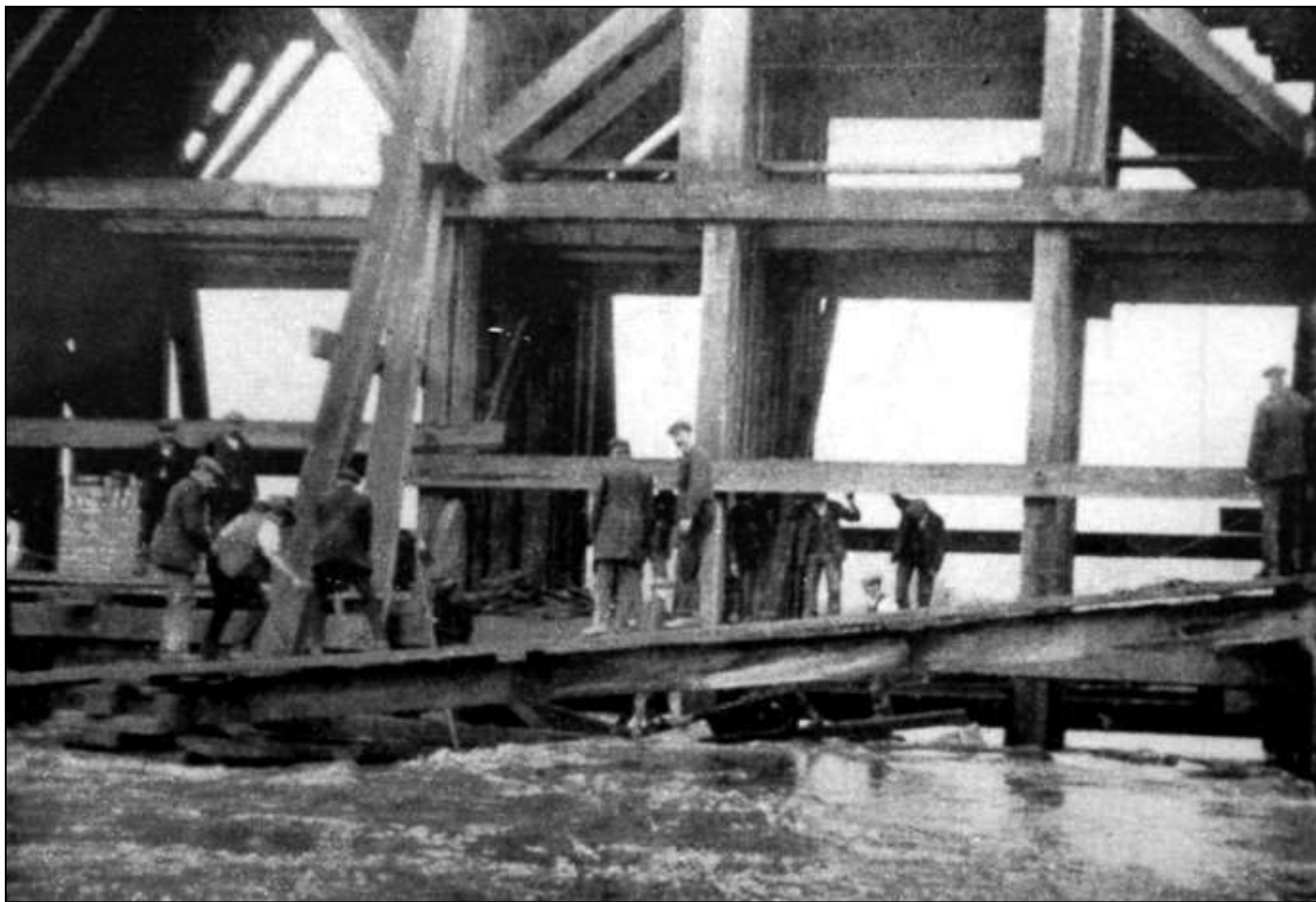
The workmen examining the timbers of the Crow Mill Viaduct under very difficult circumstances.
