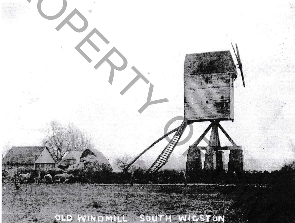
The old windmill at Crow Mill Farm, c.1900. This is a post mill where the structure is centrally pivoted and by means of the long curved pole above the ladder could be turned to face the prevailing wind. It was demolished in 1906.
