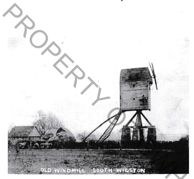
The old windmill at Crow Mill Farm, c.1900. This is a post mill where the structure is centrally pivoted and by means of the long curved pole above the ladder could be turned to face the prevailing wind.
