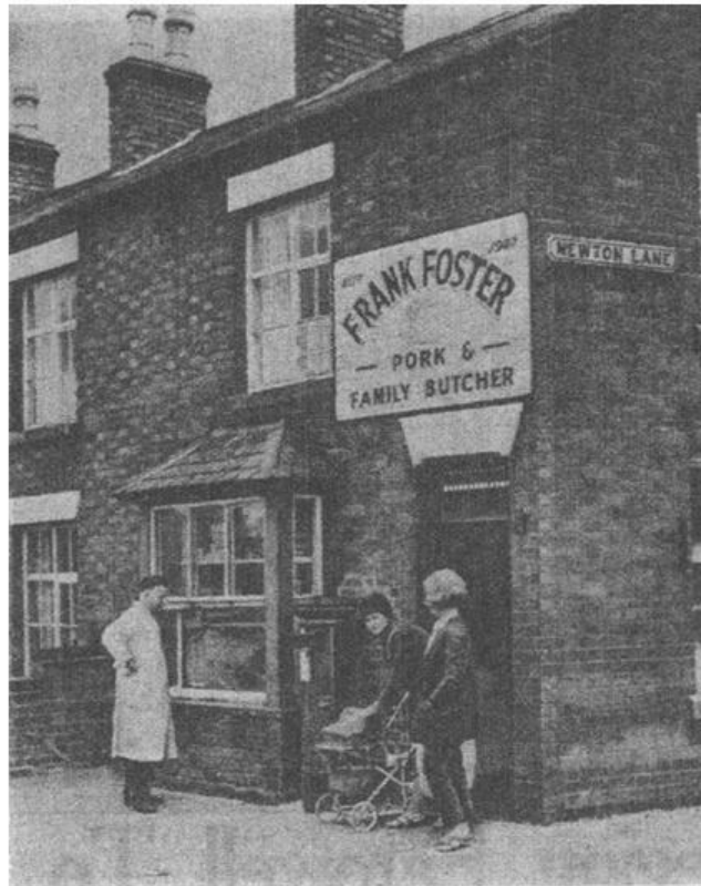
Mr Frank Foster pictured outside the butcher's shop which has stood at the corner of Newton Lane and Bull Head Street Wigston Magna for 60 years and which will be demolished in a road widening scheme
